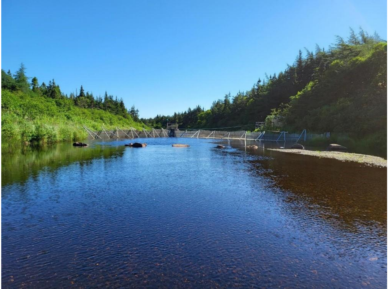
Figure 3.3 Upstream perspective of the counting fence, Come by Chance River.
